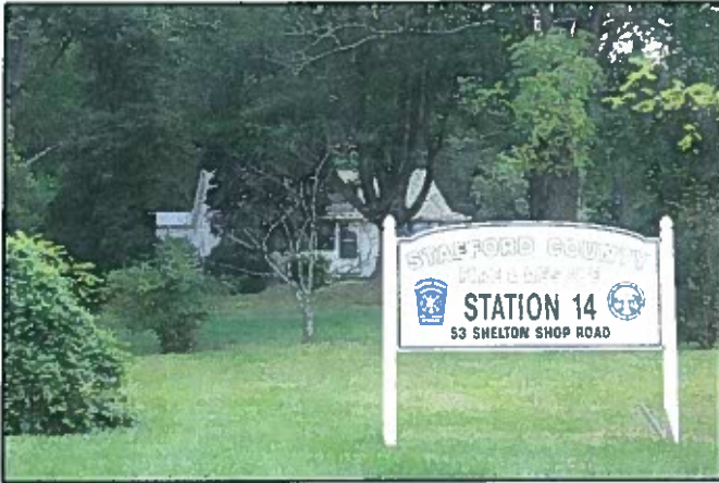
The Station 14 sign sits in front of one of Stafford's "newest" fire and rescue stations.
