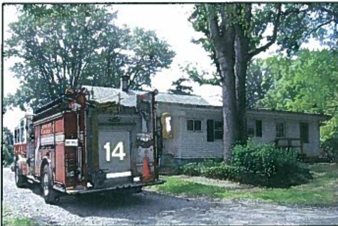
A view of the back of Fire and Rescue Station 14.
