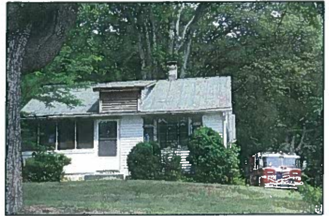
Fire and Rescue Station 14 is housed in a bungalow that was built in the 1920s.
