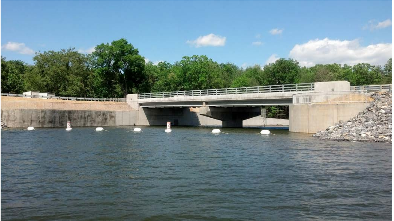
Completed Lake Holiday Spillway and bridge
