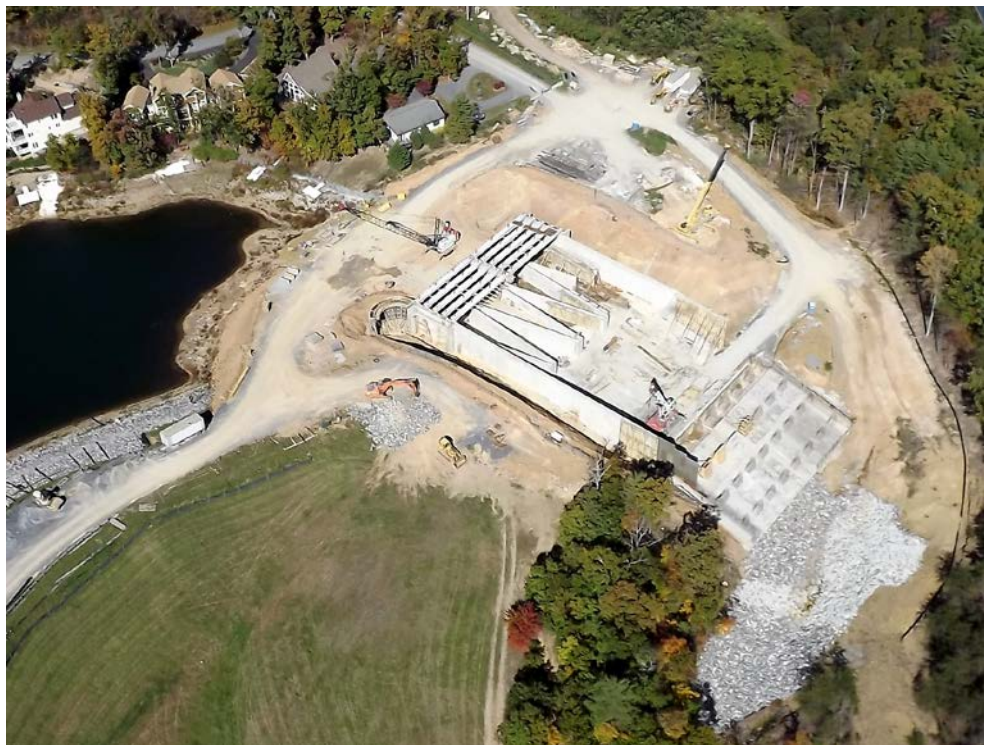
Aerial view of the spillway under construction
