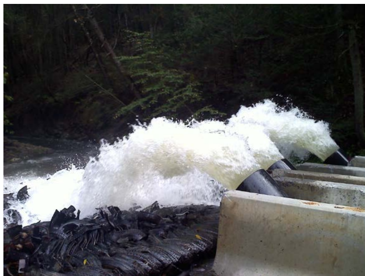
A large siphon system was used to lower the lake level over a period of weeks.
