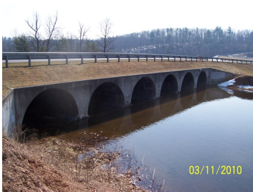
The Lake Holiday Spillway Prior to Reconstruction
