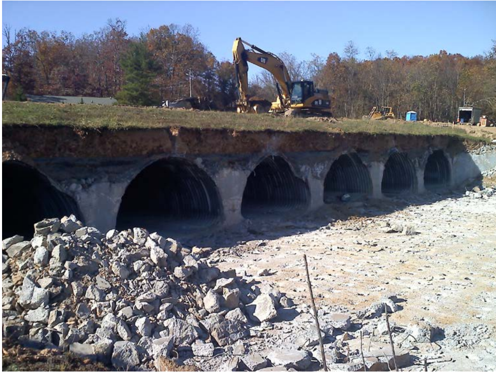
Demolition of the old spillway began in the Spring of 2011
