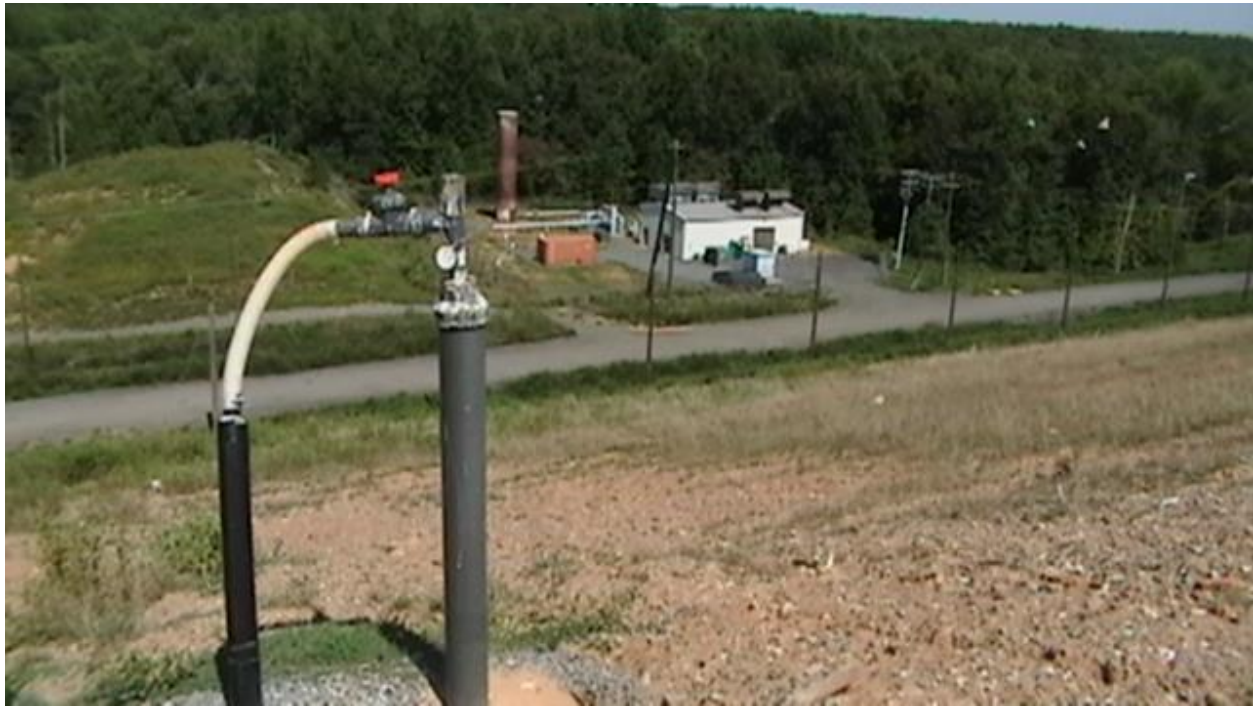
Landfill gas power plant before expansion front view.
