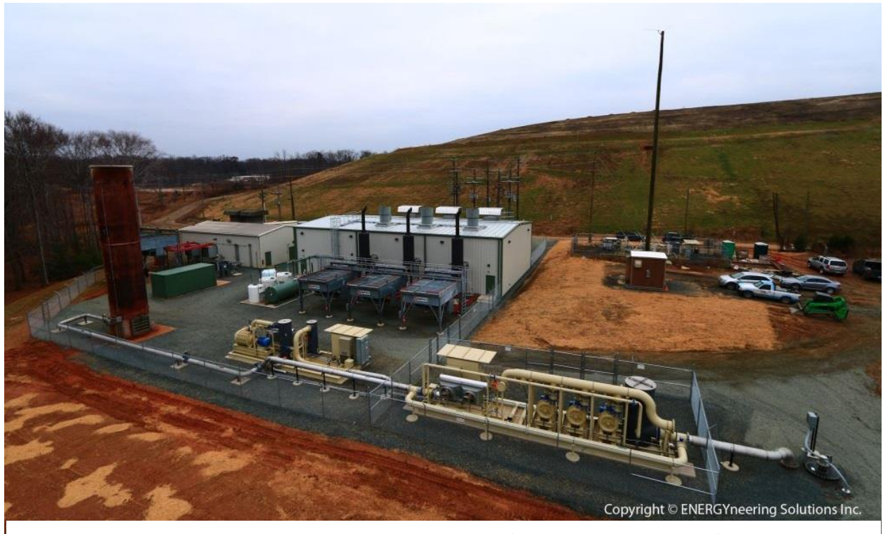
Prince William Energy showing gas skid, blower, flare, radiators, etc. after expansion.
