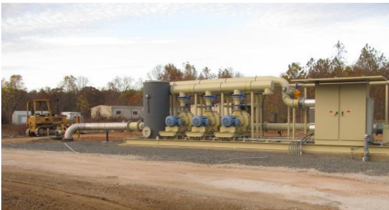
PW Facility engine blower skid
