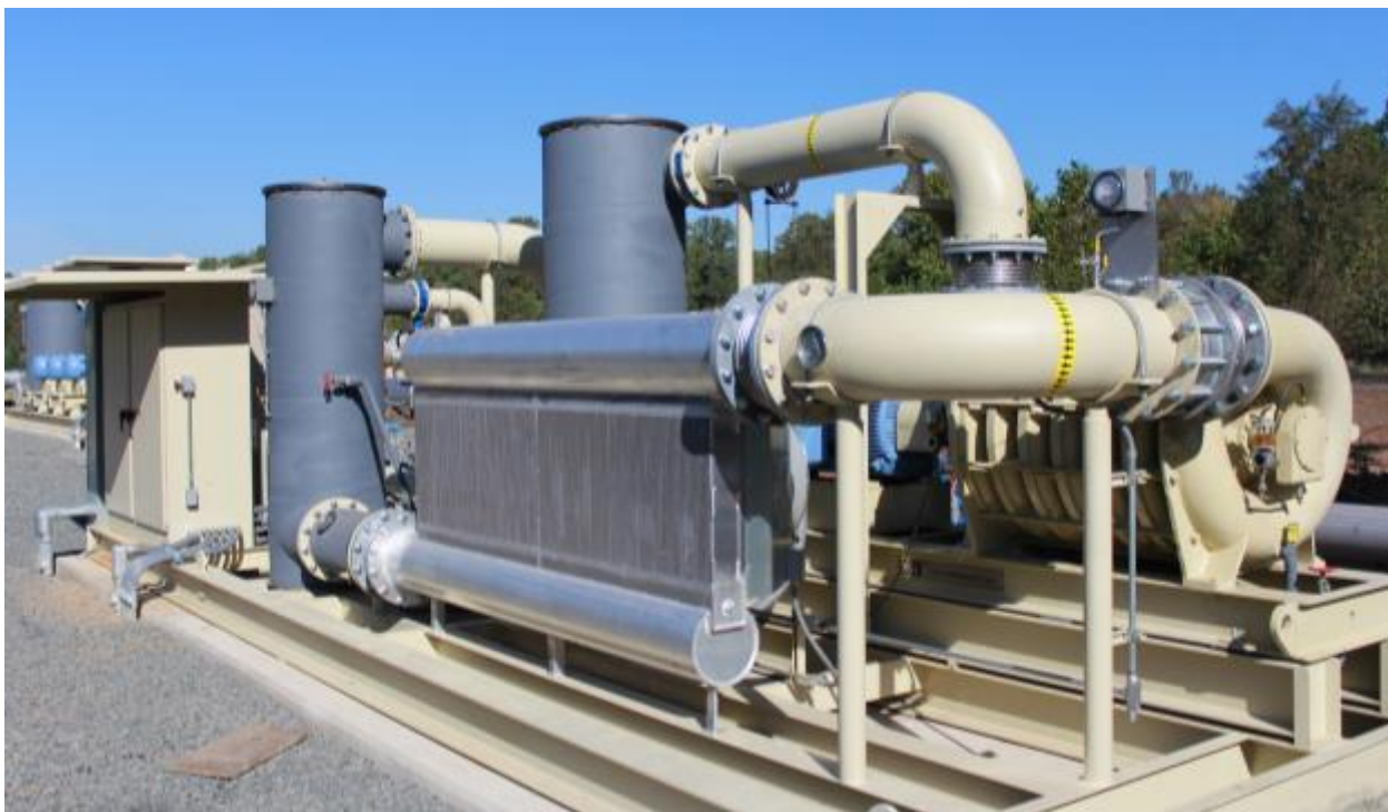
PW Facility engine blower skid
