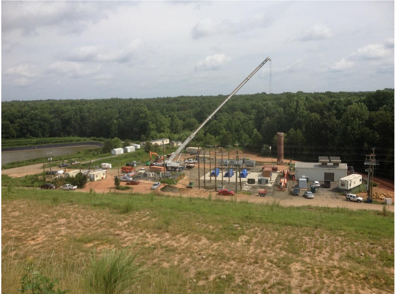
Prince William Energy Under Construction
