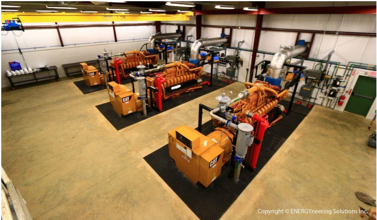
Three Caterpillar 3520 engines.
