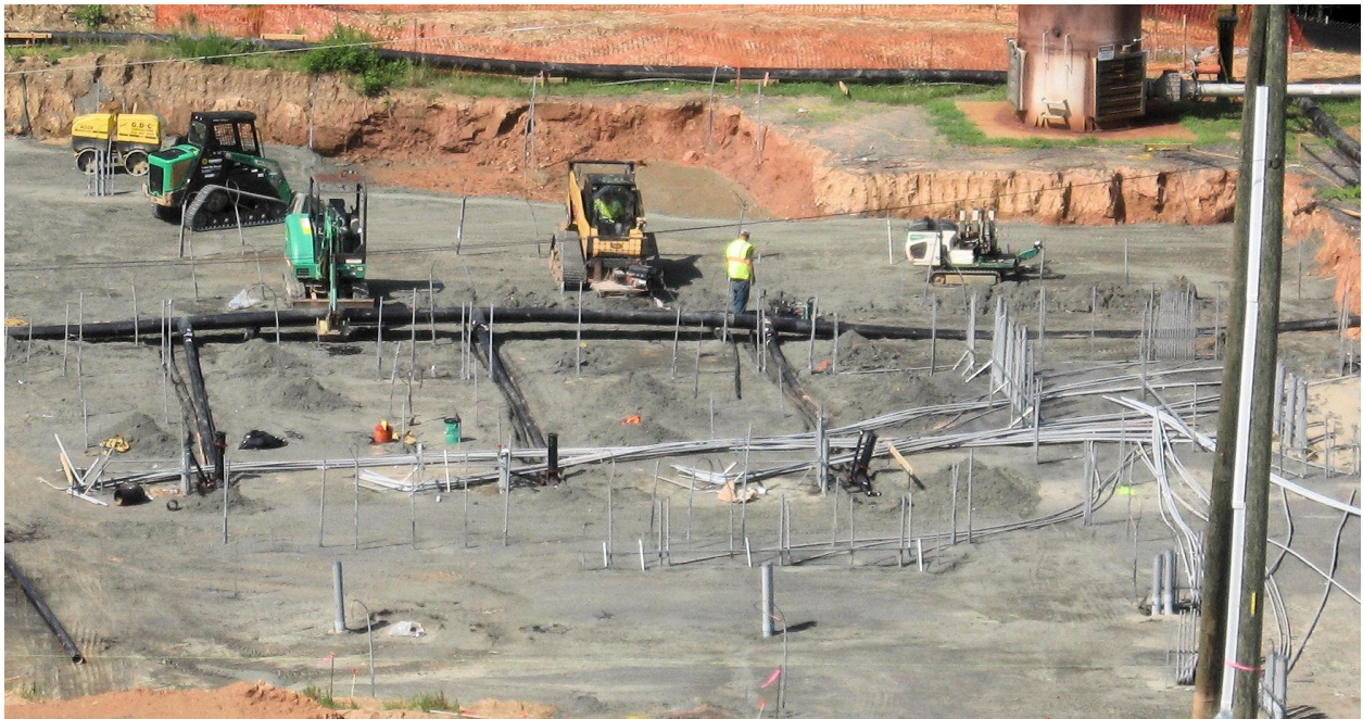
Laying conduit and high density polyethylene LFG pipes.
