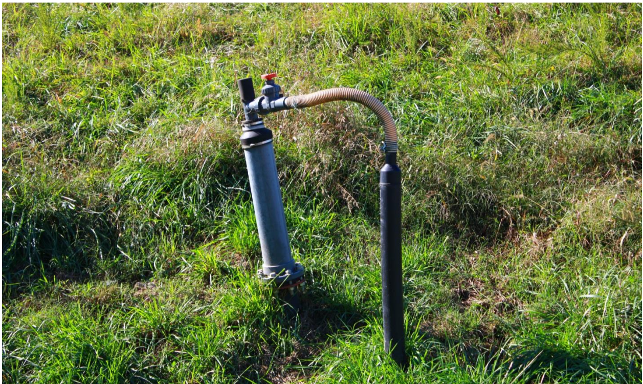
Landfill gas well.
