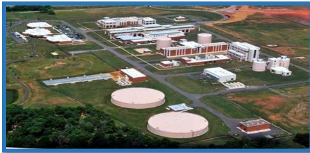
Broad Run Water Reclamation Facility
