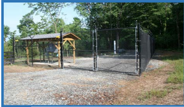
Willisville Wastewater Treatment & Disposal Facility
