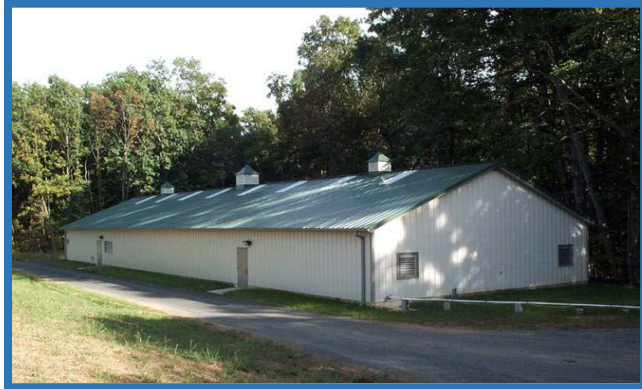
Lenah Run Wastewater Treatment Plant
