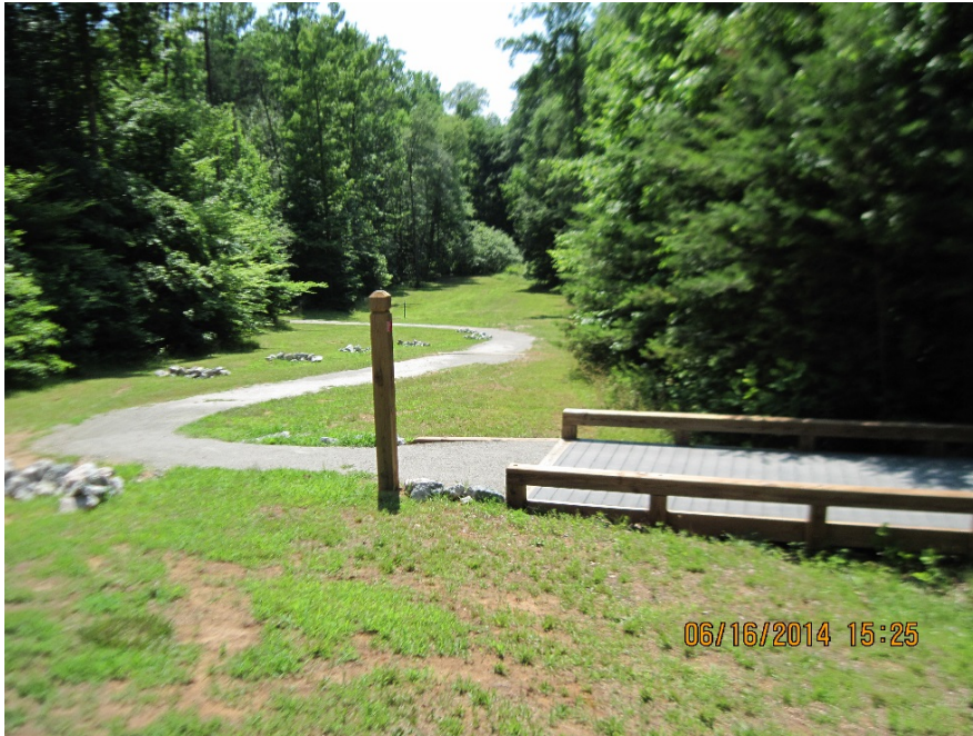
Portion of trail through Colonial Gas pipeline easement featuring newly constructed bridge and rock piles for erosion prevention
