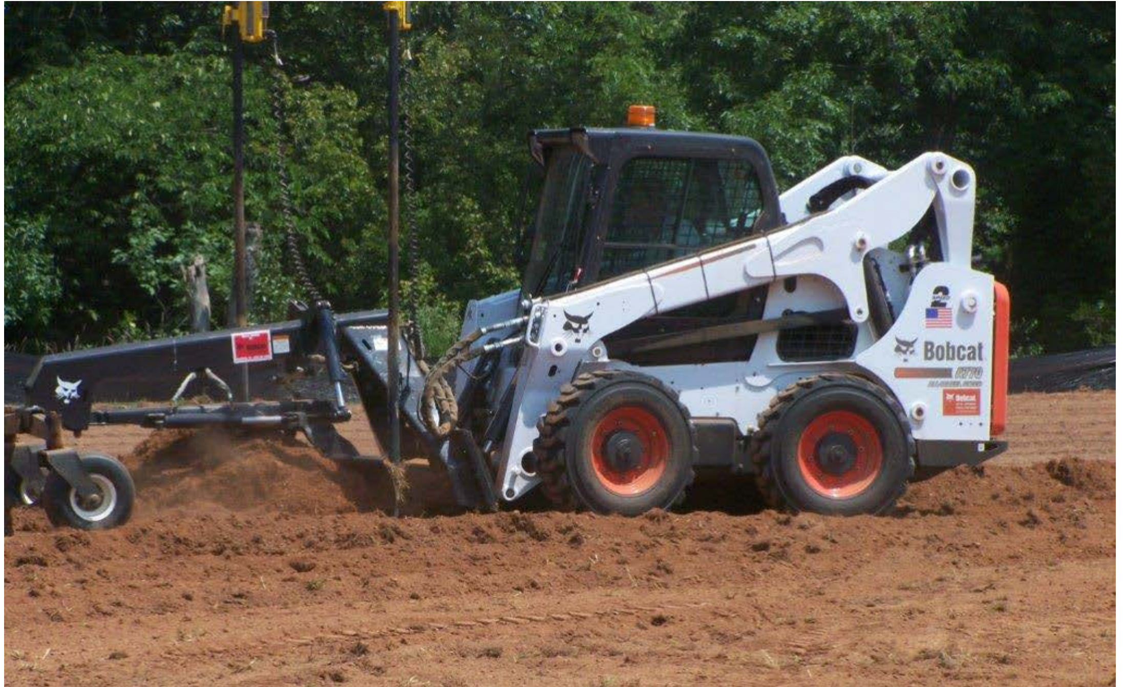
Seneca Ridge Middle School – Under Construction
