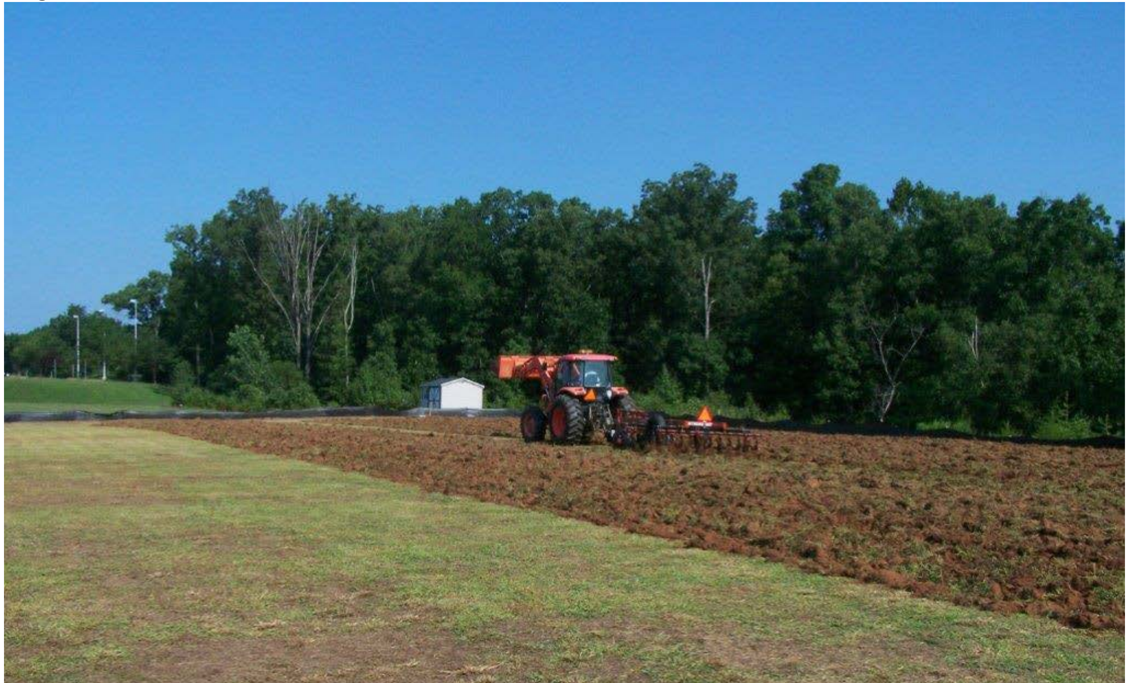
Seneca Ridge Middle School – Under Construction
