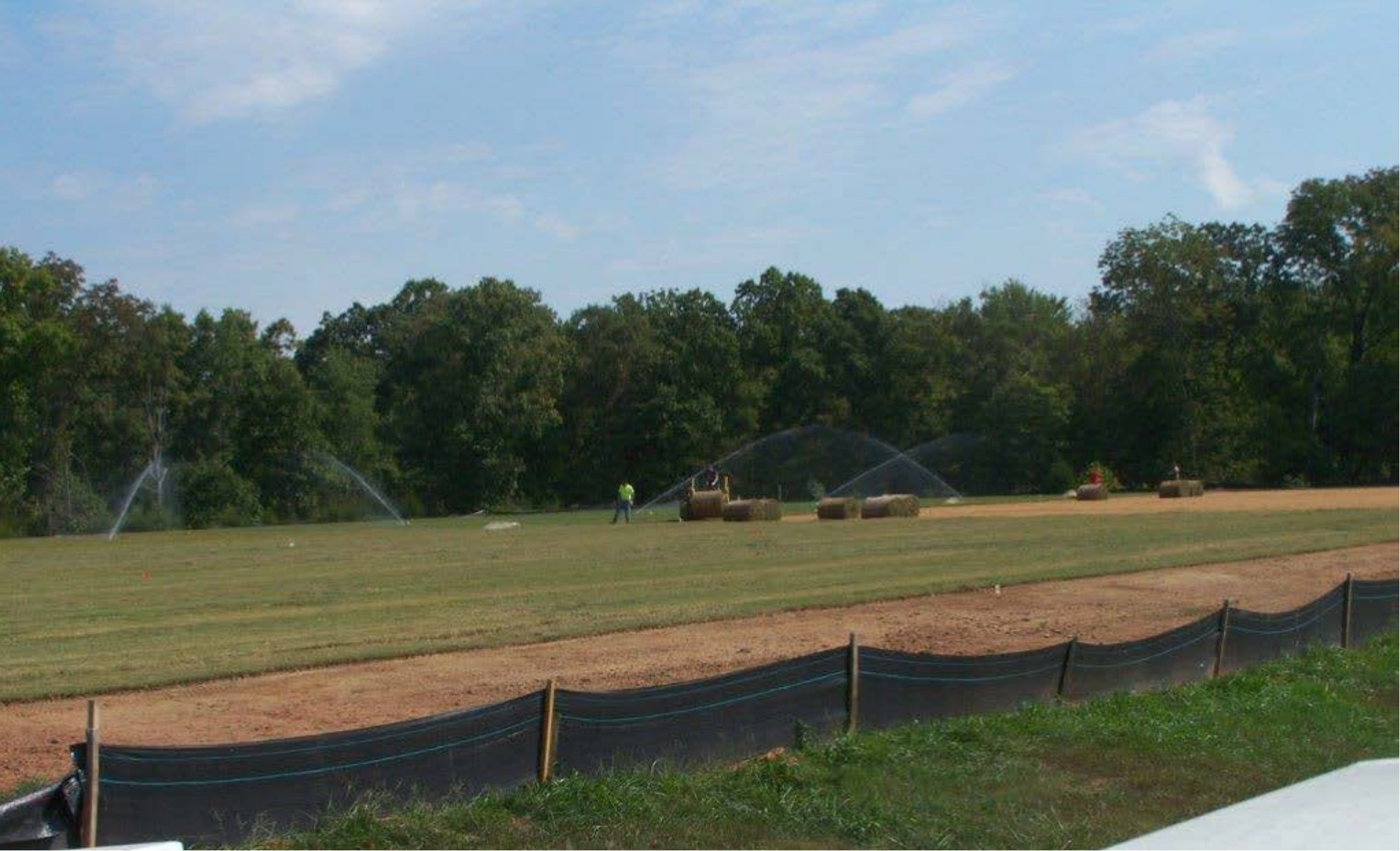
Seneca Ridge Middle School – Under Construction
