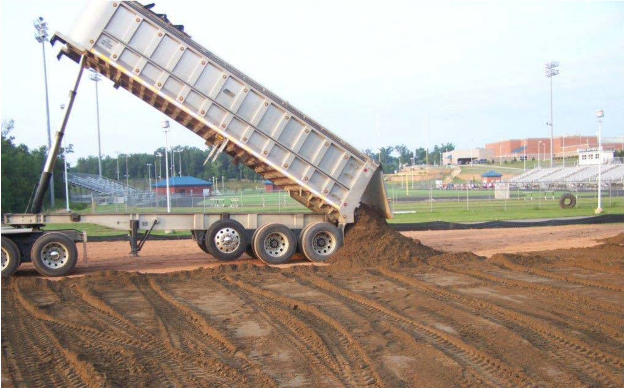
Seneca Ridge Middle School – Under Construction
